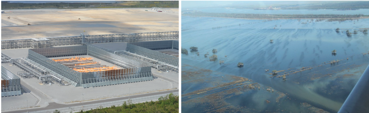
Left : Flaring at Cameron LNG after Hurricane Delta in 2020. Right : Flooding at Global's Plaquemines LNG site after Hurricane Ida in 2021. Photographs by Healthy Gulf.
